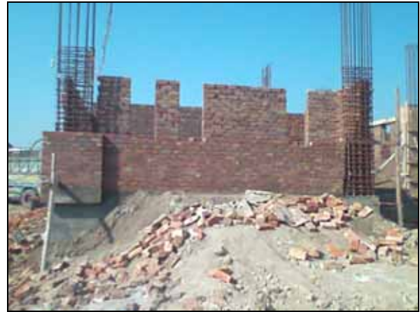
Steel cutting, bending and binding work on site
