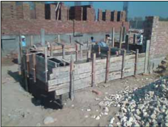
Shuttering work in progress
