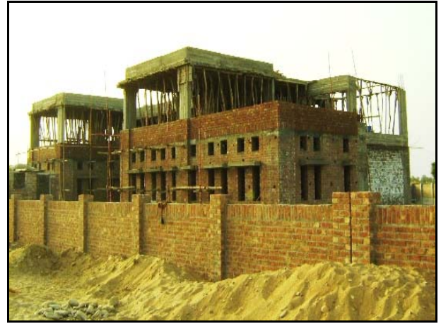
Brick masonry of the school completed
