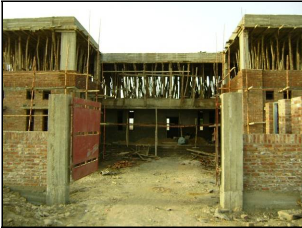
Front view of the school under construction
