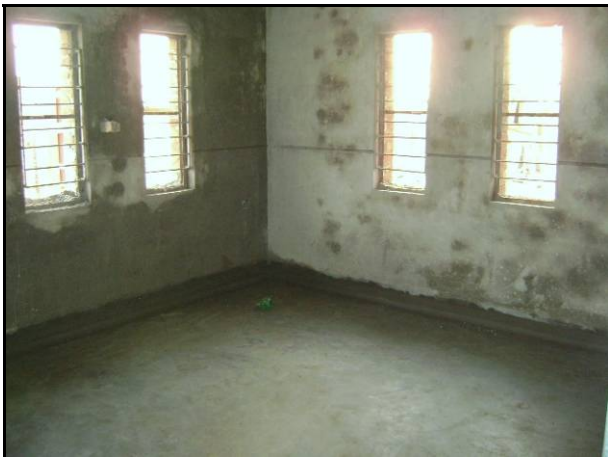
Inside view of the classroom under construction
