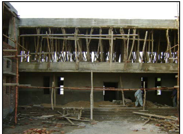
Roof slabbing on first floor completed
